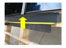
Fix the lower part to the left with another wood screw  $4.5 \times 35$  mm.
