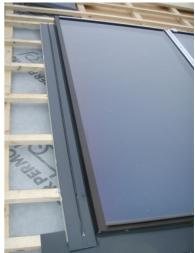
Hook in the TOP-LEFT CORNER part outside at the side flashing, turn down and slide upwards.
