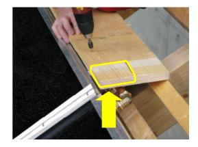
Put the side part of the flashing to the lower corner and place it parallel to the lateral squared timber of the collector.
