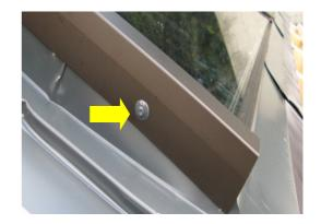
Engage the upper parts of the flashing diagonally into the sheet fold in a number corresponding to the number of collectors to be mounted, and shift the flashing together (observe the control measure of 500 mm).
