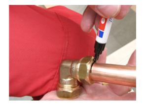
Connect the collectors hydraulically as per photo. Snug-tighten the screwed connection and then tighten it with a complete turn (mark nut and fitting).
