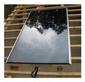
Fix in place the collector on the mounting angle with 4 Spax screws 4.5 x 30 mm.
