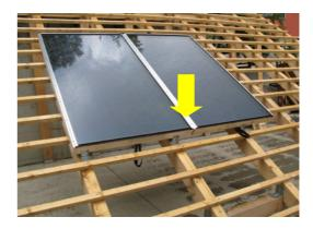
The collector is fastened to the mounting angle with 4 Spax screws  $4.5 \times 30$  mm.
