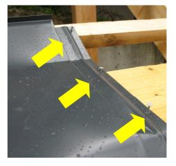
Engage the upper parts of the flashing diagonally into the sheet fold in a number corresponding to the number of collectors to be mounted, and shift the flashing together (observe the control measure of 500 mm).
