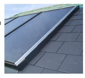
**26)**Fix the right and left covering strip with 3 wood screws 4.5 x 35 mm
