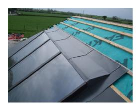
Put the cover rail, as shown in the photo, between the collectors and lock them by slightly knocking with the palm of your hand. Align the cover rail flush with the collector by means of a hard rubber hammer.
