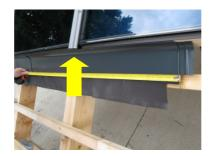
Fix the lower part to the left with another wood screw 4.5 x 35 mm.
