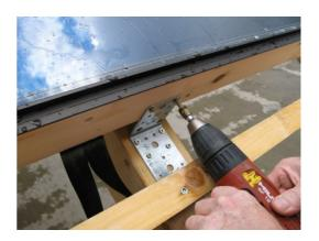
The second collector is fixed at the RIGHT SIDE with 3 Spax screws 4.5 x 70 mm.
