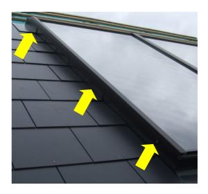
**27)**Put in place the wooden support wedge. If required, mount an additional roof batten as a support.
