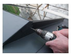
**ATTENTION:** The flashingmust be engaged in the upper profile of the collector!
