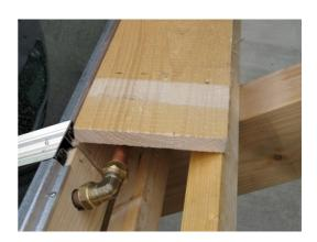
Screw all wooden support wedges with 2 Spax screws  $5.0 \times 120$  mm and 2 Spax screws  $4.5 \times 70$  mm each to the roof battens.
