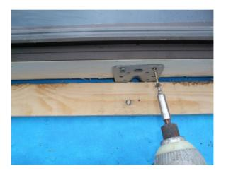
Fix the collector in place at either side with 3 Spax screws 4.5 x 70 mm.
